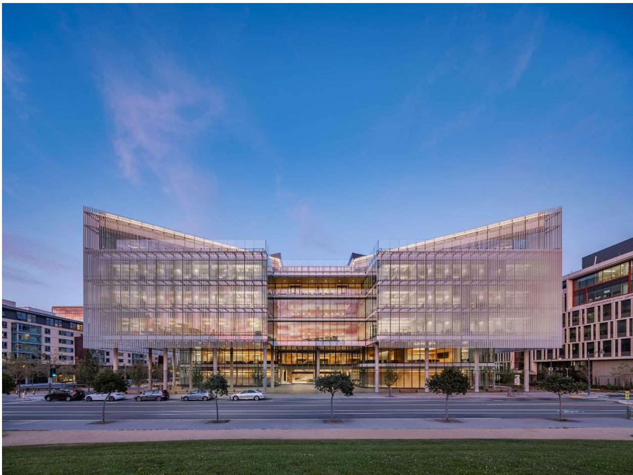
Photo © Tim Griffith
