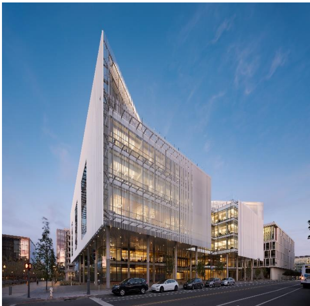
Photo © Tim Griffith
