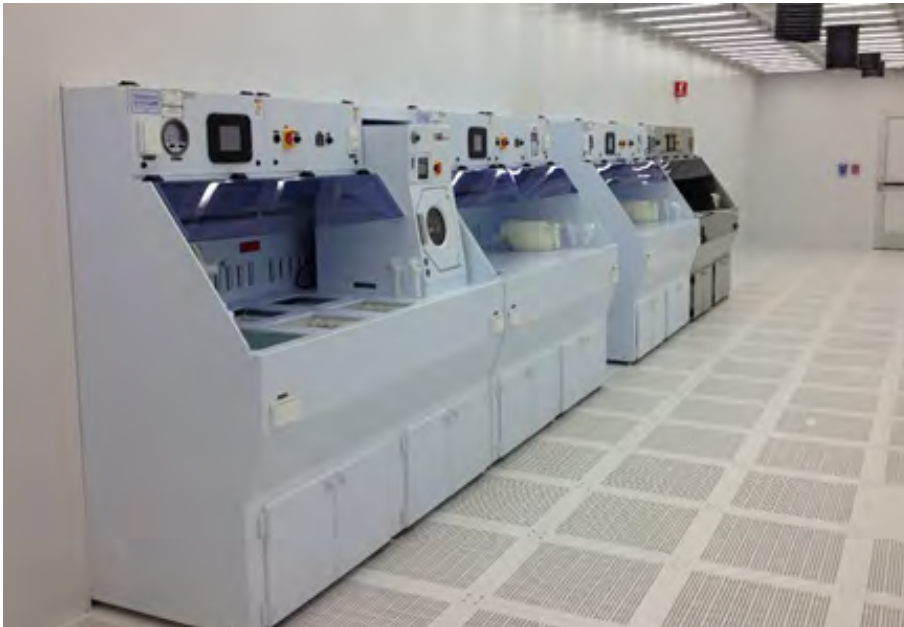
Figure 33 Wet Process Workstations
