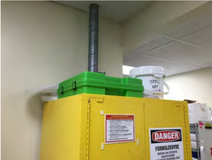
Figure 34 Ventilated Flammable Gas Cabinets
